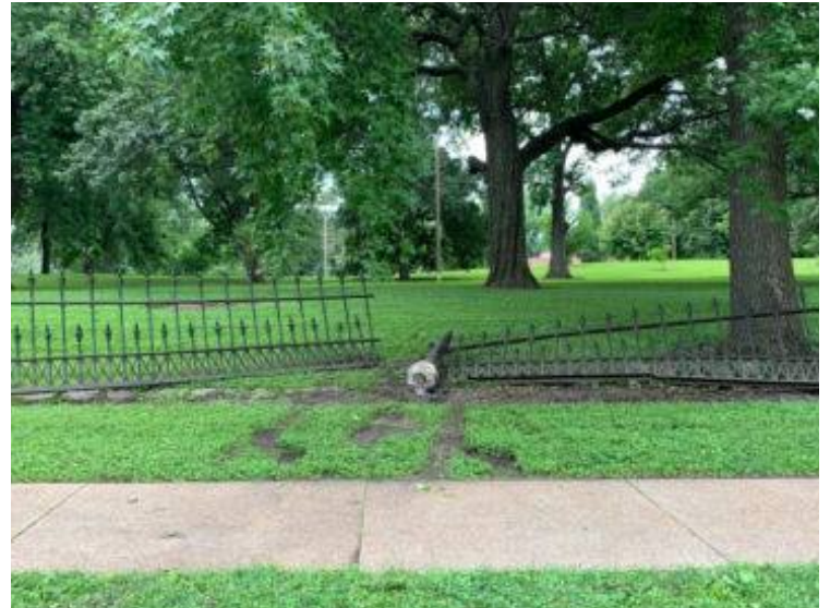
Section of fence along Park Avenue after being hit by a car.
