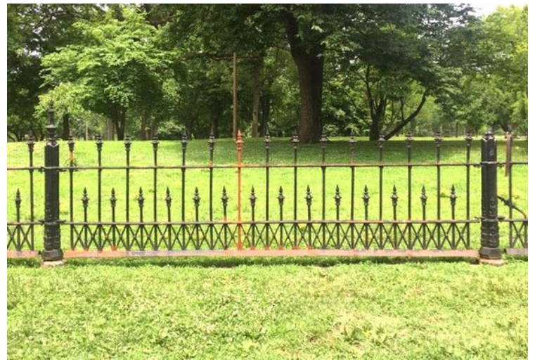
Section of fence along Lafayette Avenue after being repaired this June.
