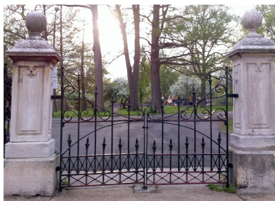
One of the park entrance gates in need of repair.
