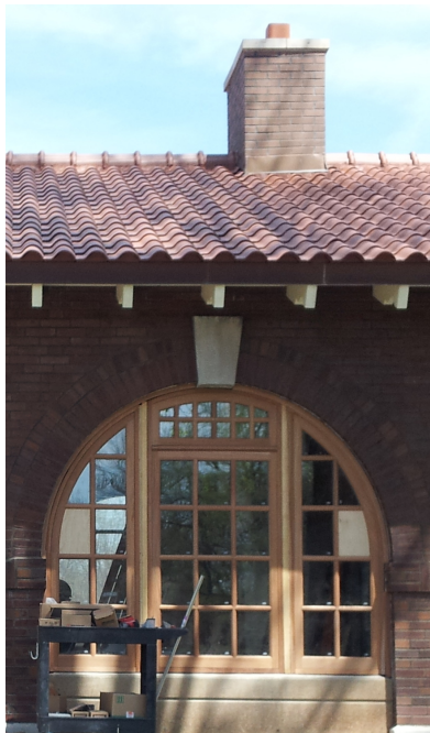
New windows as seen from the exterior.
