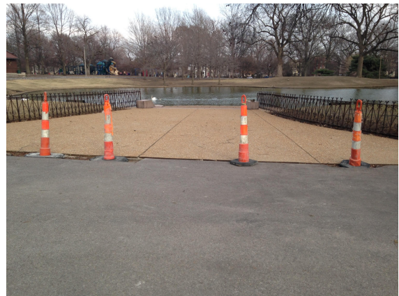
Repaired concrete pad near the lake in Lafayette Park.
