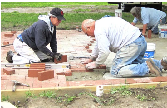
Ron Taylor, Tim Delahanty and Larry Dodd lay bricks.
