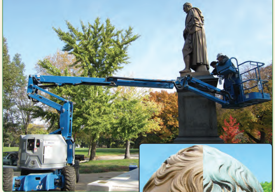
Benton Monument undergoing conservation, October 2014
