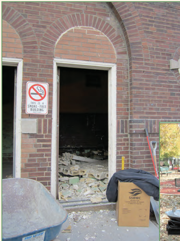
Demolition of the old woman's restroom.
