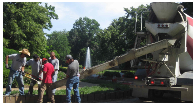
A crew constructing one of the cement curbs.
