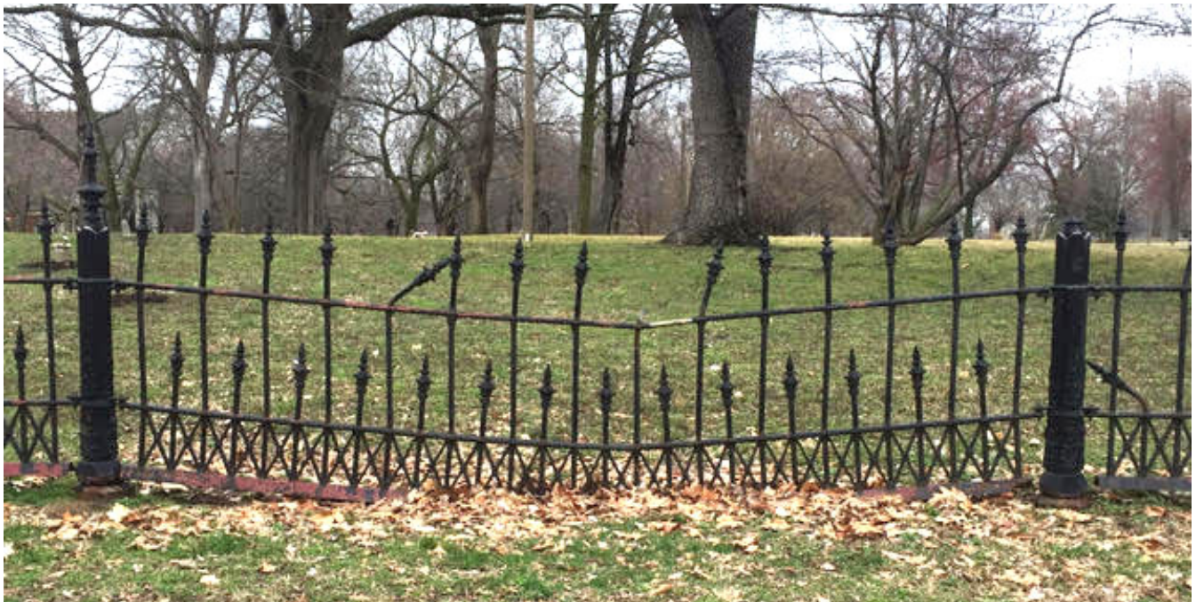
Fence section crumpled by a fallen tree near Lafayette and Missouri that will be replaced.
